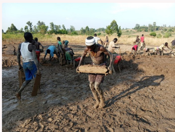
Youths of Alibajiako Village, Terego District, laying bricks for the Home Learning Centre's upgrade
